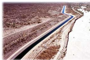
Hayden-Rhodes Aqueduct, Arizona Bureau of Reclamation
