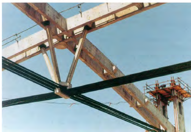
Figure 4. The roof structure of sports hall Belgrade Arena (1992) – two-chord externally prestressed reinforced concrete girders, spans 132.7 and 102.7 m, covering the area of 15000 square meters
