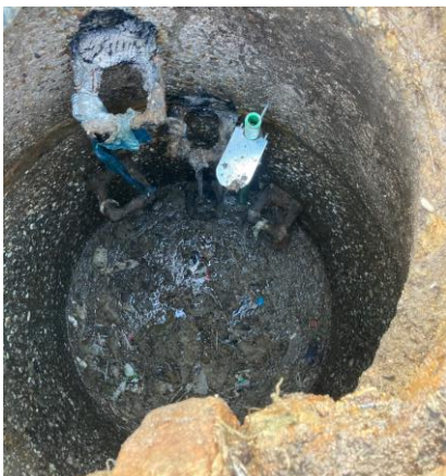
Slika 1. Stanje u Š SP2 i Š SP3 , tokom montaže opreme Figure 2. Manholes Š SP2 and Š SP3 state in regular operation
