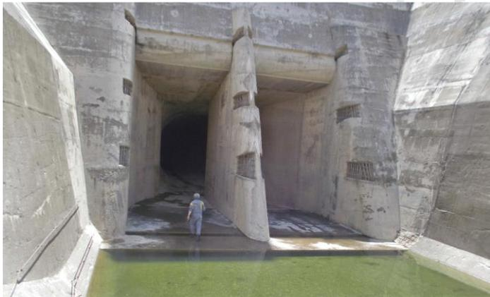
Inlet structure with flow divider
