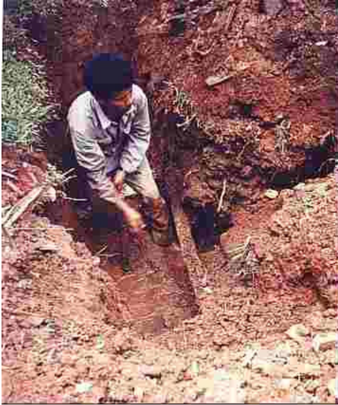
Figure E-2 Excavation by hand
