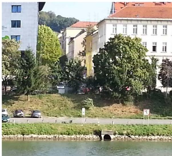
Figure 3. Combined sewer system outlet at the Drava River, partially surcharged what often occurs even for medium and low intensity rainfall events
