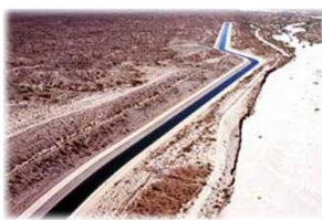
Hayden-Rhodes Aqueduct, Arizona. Bureau of Reclamation
