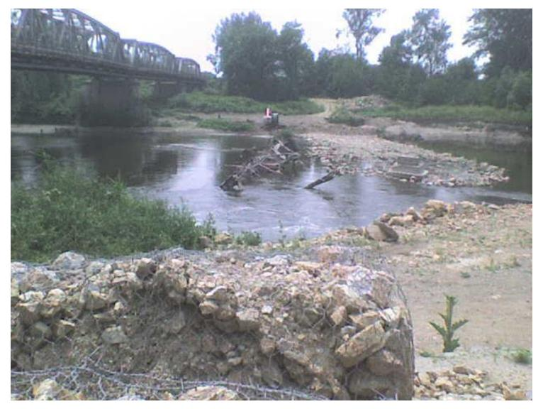
Overflow at sill which was noticeable but regular during first year after construction works at the end of year 2008.
