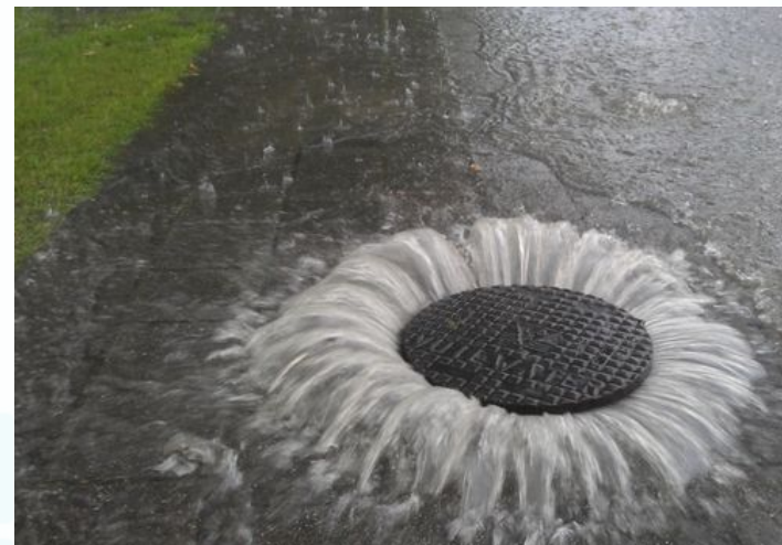
Sewer system flooding
