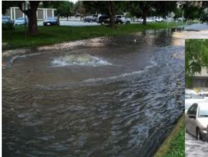
1- Surcharge event in sewer system of Auckland, New Zealand, 2009
