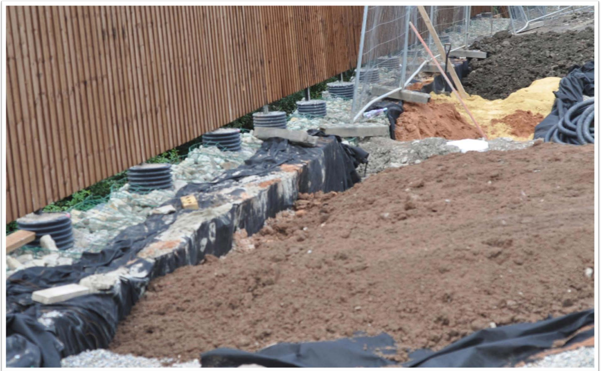
Gravel covered with soil up to finished garden level
