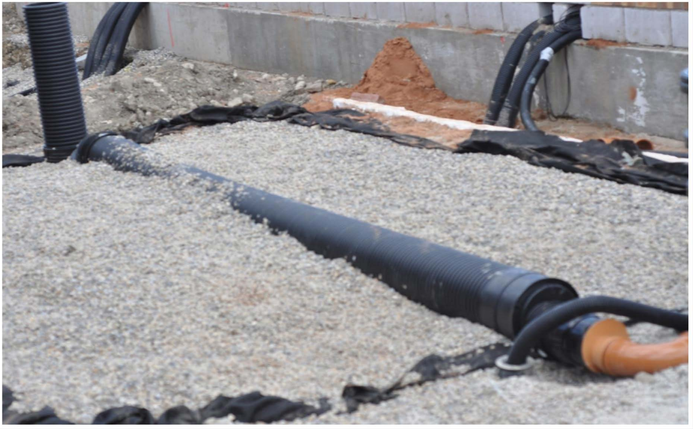
Covering sand with 750mm deep gravel for rainfall drainage
