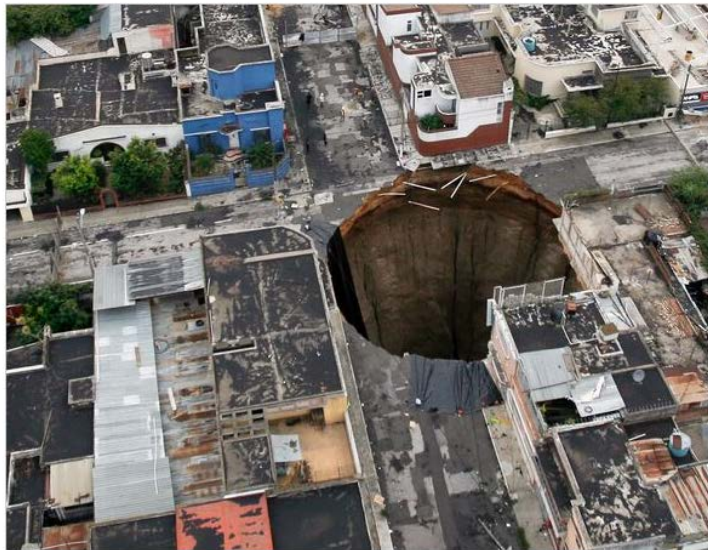
The sinkhole appeared Sunday in downtown Guatemala City, swallowing a three-story building.
