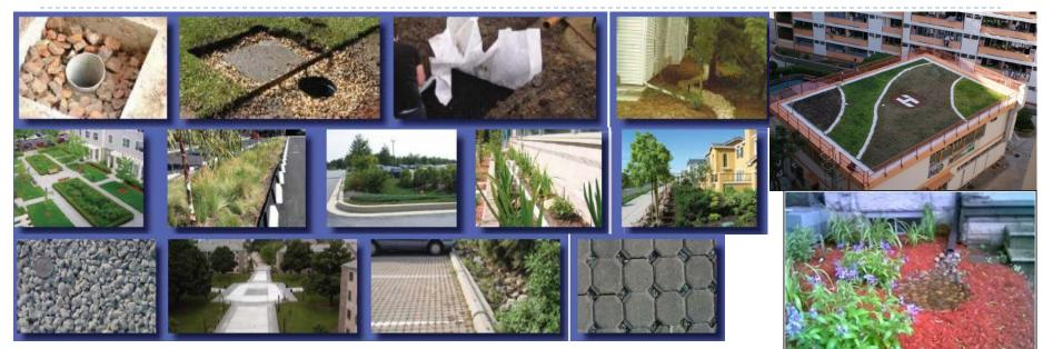
Soakaway pit, dry well, rain harvesting, downspout disconnection, greenroof, bioretention cell, porous pavement, 17 combinations
